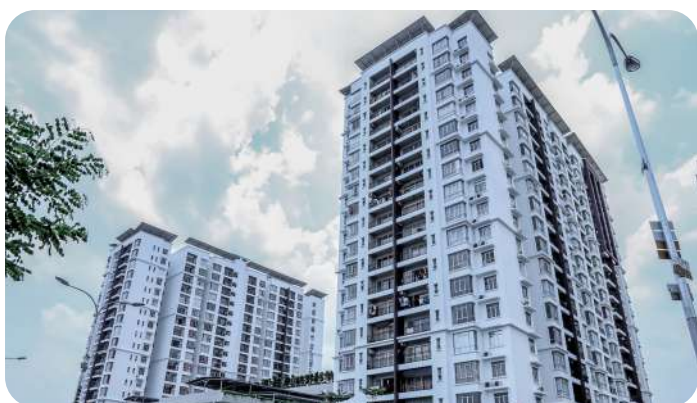
1120 Park Avenue Condominium
